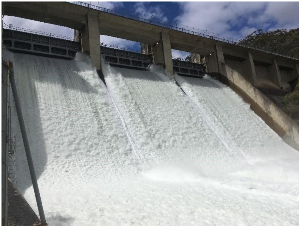
Figure 6: Lake Eildon spillway at 38,000 ML/day (15 October 2022)
